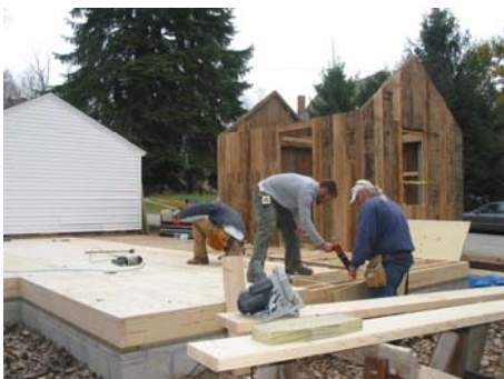
Work on the Library Expansion is proceeding
