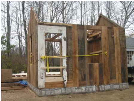
The John F. Williams Law Office under reconstruction
